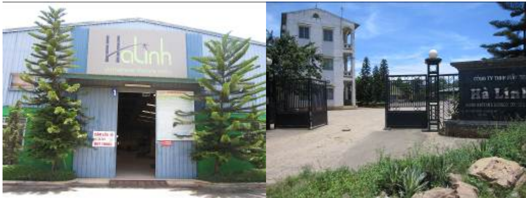
Outside's company and a workshop
